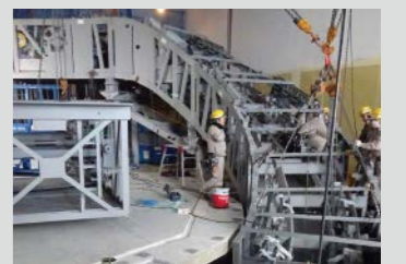
Truss installation work
