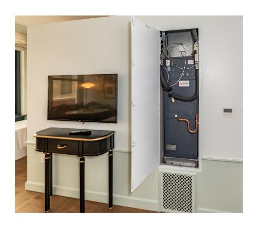
Multi-Position Ducted Air Handlers (PVFY) throughout the hotel and six Ductless Indoor Units (PKFY) in their audio-visual rooms. The heating and cooling system is controlled through the AE-200A Centralized Controller.
