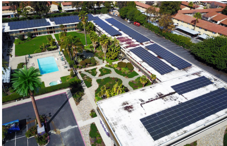
Ramada Silicon Valley recently installed a 269 kW photovoltaic system with 996 Mitsubishi Electric Diamond Premium modules.
