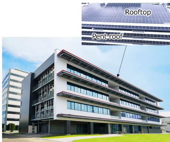
SUSTIE ZEB test facility
