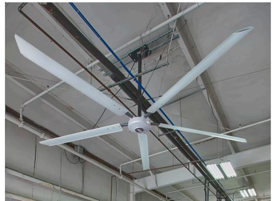
Hunter Fan provides high-velocity, low-speed (HVLS) fans for industrial and commercial use.
